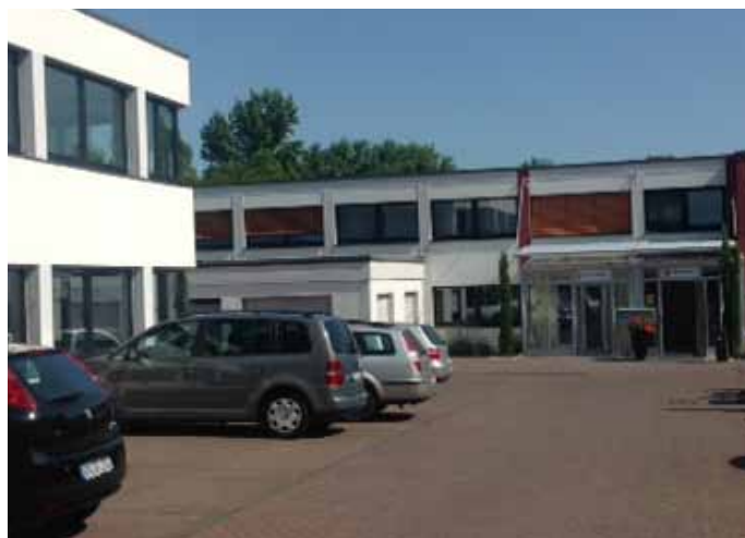
Office Complex on Heilsbach Street in Bonn-Duisdorf
